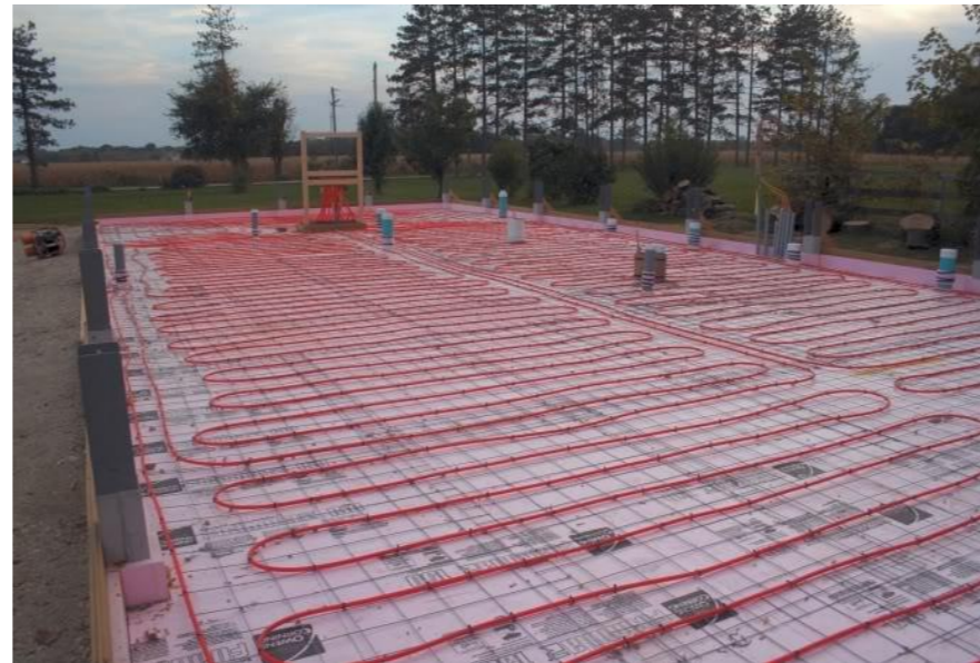
Figure 18 – Underfloor heating PEX piping
