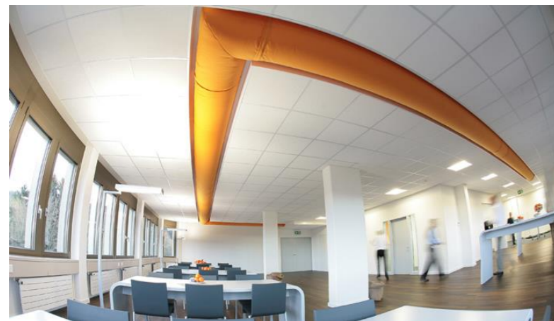
Figure 26 - Fabric duct installation example
