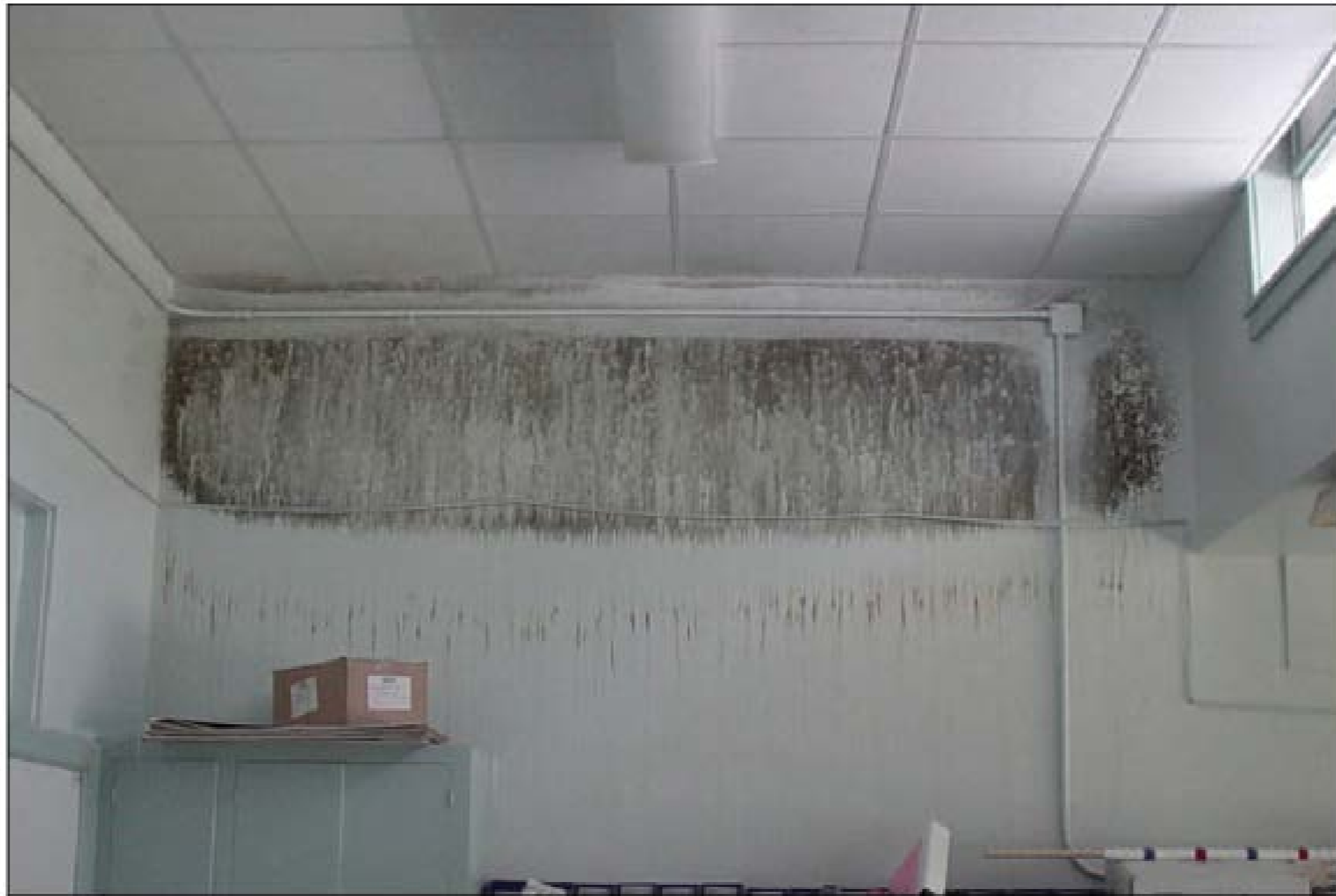
Photograph 1: Mold growth on classroom wall after 72 hours.
