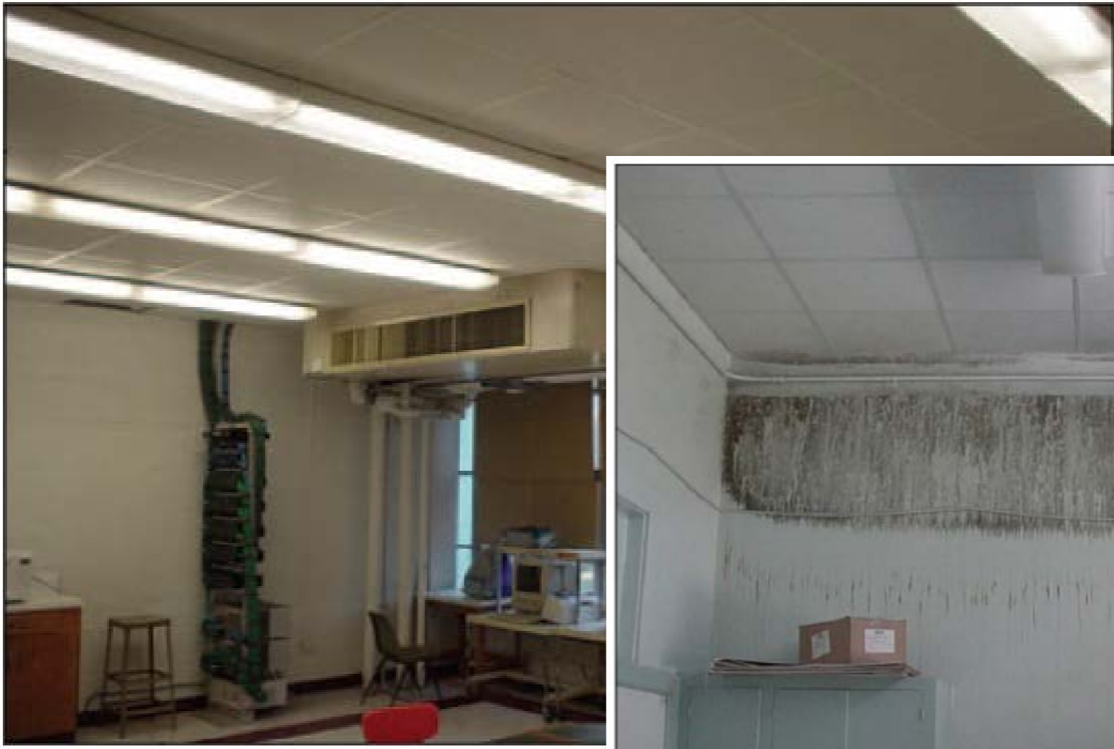
Photograph 1: Mold growth on classroom wall after 72 hours.
