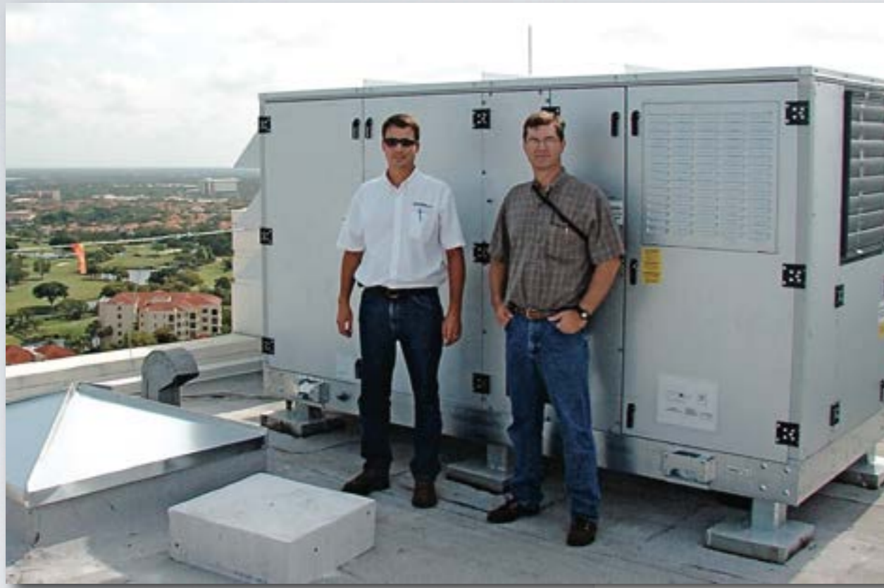
DOAS unit for Ventilation & Dehumidification
