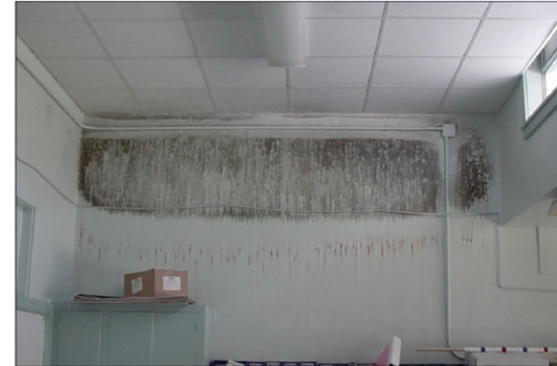
Photograph 1: Mold growth on classroom wall after 72 hours.
