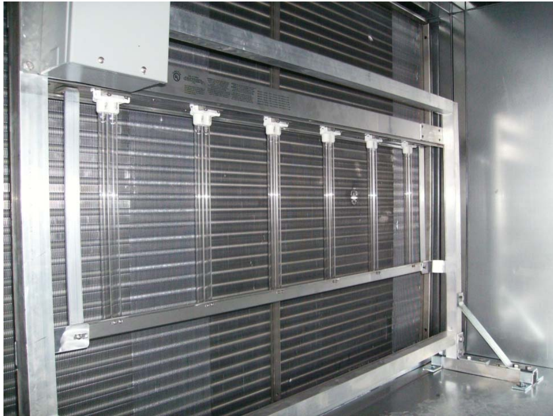
Downstream coil surface/air installation
