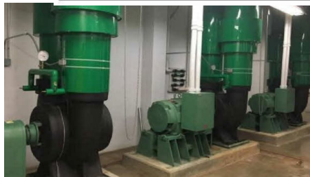
Chilled Water Pumps
