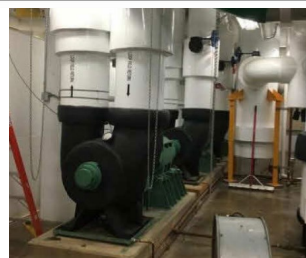
Ground Loop Pumps
