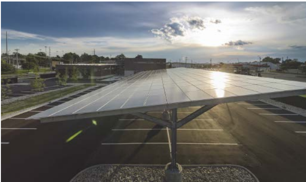
Figure 5-67 (RE5) Canopy-Mounted PV System Used with Permission from CMTA, © Dish Design
