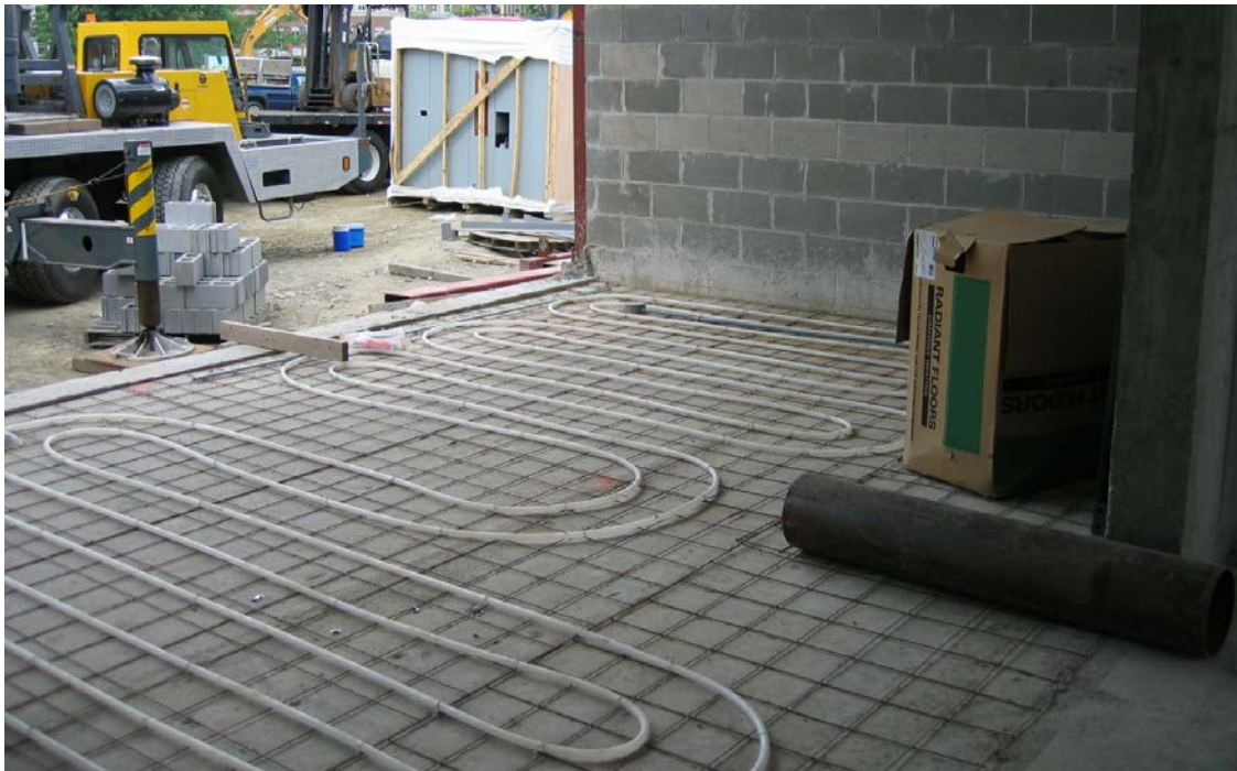
Figure 5-53 (HV19) Radiant System in Multifamily
