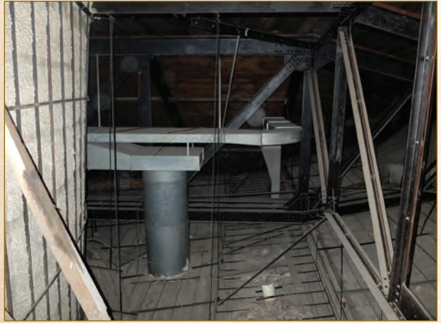
Figure 10 Ulster Performing Arts Center. This shows a typical condition in many early 20th century theaters, with plaster ceilings hung from metal strap hangers, making major changes often difficult to achieve without potential risk to historical finishes. Source: DLR Group
