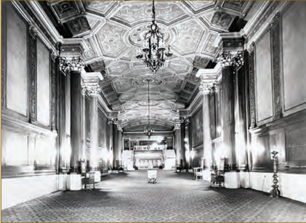
Figure 9 Ohio Theater Lobby. This series of photos shows the lobby (Top) in its original condition; (Center) after a later renovation; and (Bottom) after its recent historic restoration. Source: DLR Group
