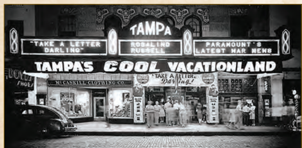
FIGURE 11 Tampa Theater. (Top) The first air-conditioned commercial building in Tampa advertised its indoor environment as a Cool Vacationland. Source: Cinematreaasures.org. (Bottom) The recently restored theater, including new seating, upgraded lighting and reconfigured return air distribution. The original installation utilized hundreds of floor-embedded mushroom return air devices. These often became difficult to maintain, if a drink was spilled on the floor. Source: DLR Group
