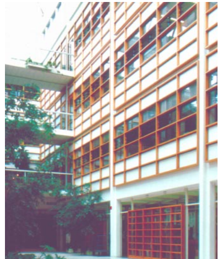
Figure 5: Atrium at Gateway House.
