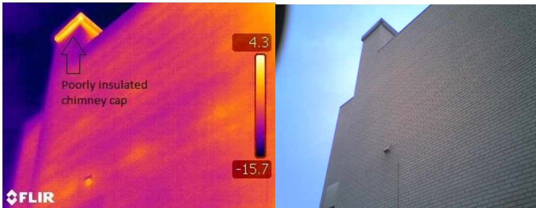
FIGURE 3: INFRARED PHOTO: POORLY INSULATED CHIMNEY CAP
