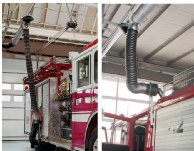
Figure 11 - High-level and Low-level Tailpipe Connection
