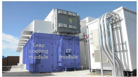
Figure 5 Air-side economized modular data center with evaporative cooling module.
