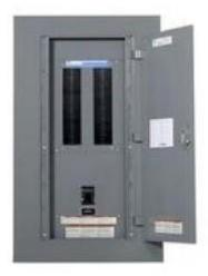
Figure 22 Photo of typical data center wall-mounted panelboard.
