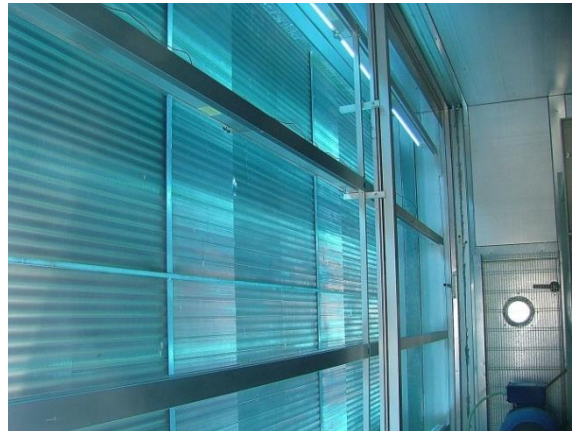
Figure 1. UVGI System Design
