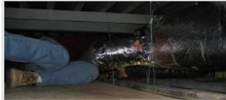
Figure 4.3-C System Location Limits Access
