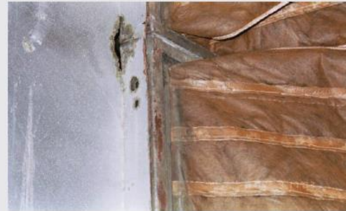
Figure 7.5-J Corrosion Penetration within an Air Handler
