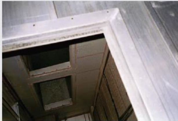
Figure 7.5-I Eroded Gasketing on Filter Access Door
