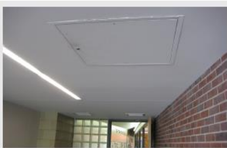
Figure 4.3-A Access Door to Systems
