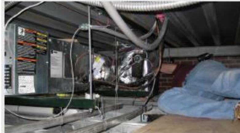
Figure 4.3-D All System Components not Readily Accessible
