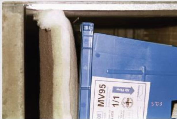
Figure 7.5-H Fallen Filter with Substantial Visible Gap
