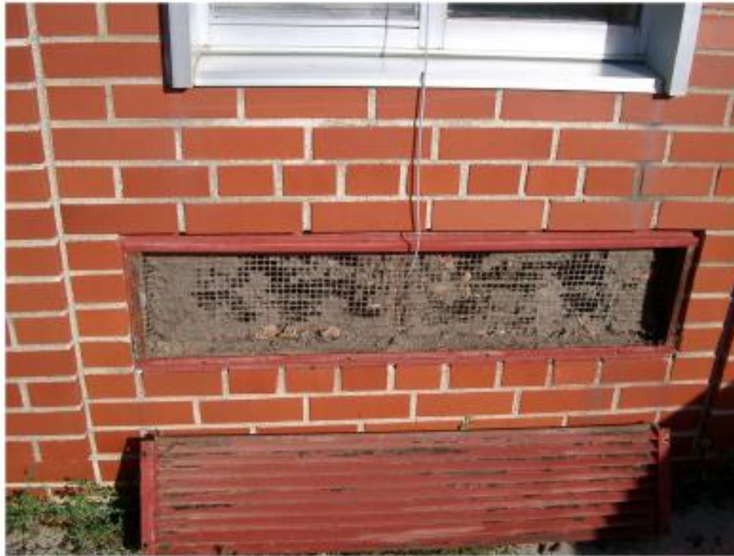
Figure 1.5-H Mismatch between the Amount of Equipment to be Maintained and O&M Staffing Levels—Clogged Outdoor Air Intake on One of Many Classroom Unit Ventilators in a School Photograph courtesy of Mark Hancock.
