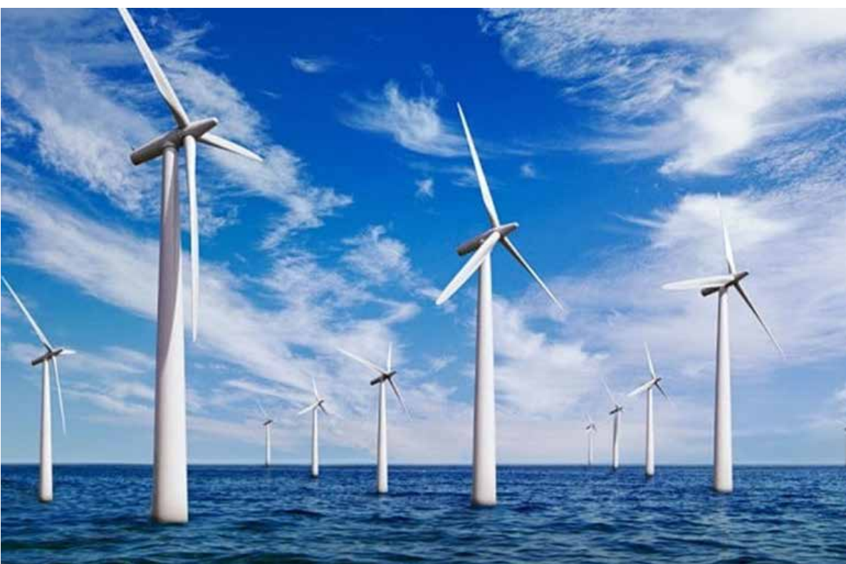
Offshore Wind Energy: One 91m Diameter Turbine Peak: 1,142 kW Annual: 10,000,000 kWh
