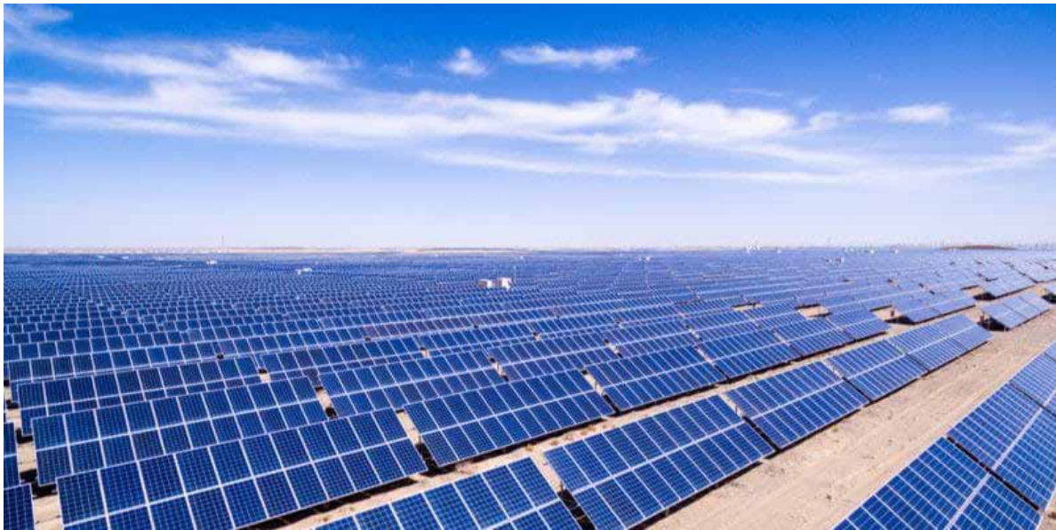
Solar Energy: 3,735 m2 2-axis tracking array Peak: 561 kW Annual: 1,250,000 kWh
