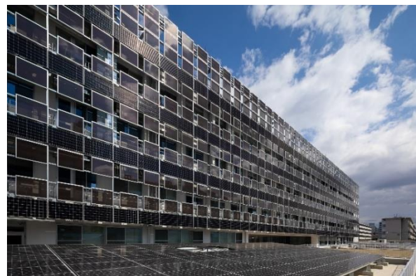
Photo 1 Ground View from South-West
