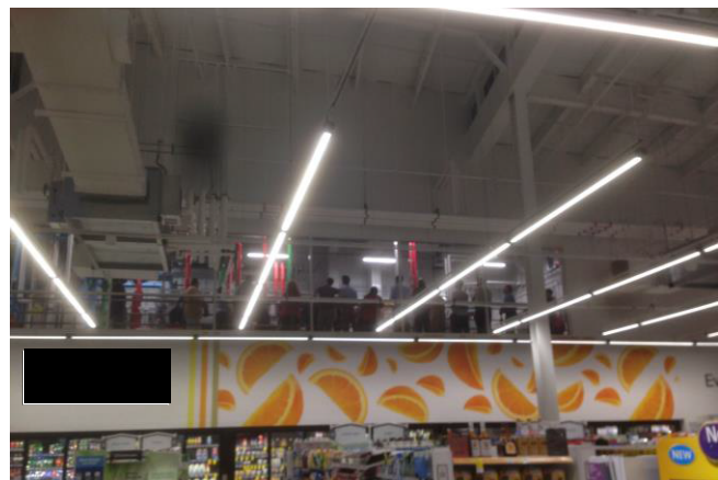
Figure 4 - Mechanical Room with a Tour Group
