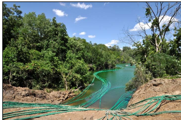
Figure 3: Installation of Pond Loop Condenser Water Piping.
