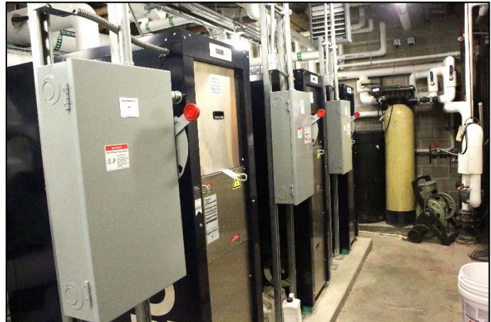
Figure 2: Water Source Heat Pumps.
