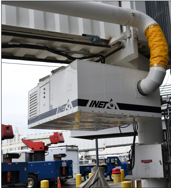
Gate PC Air unit, telescoping duct and hose
