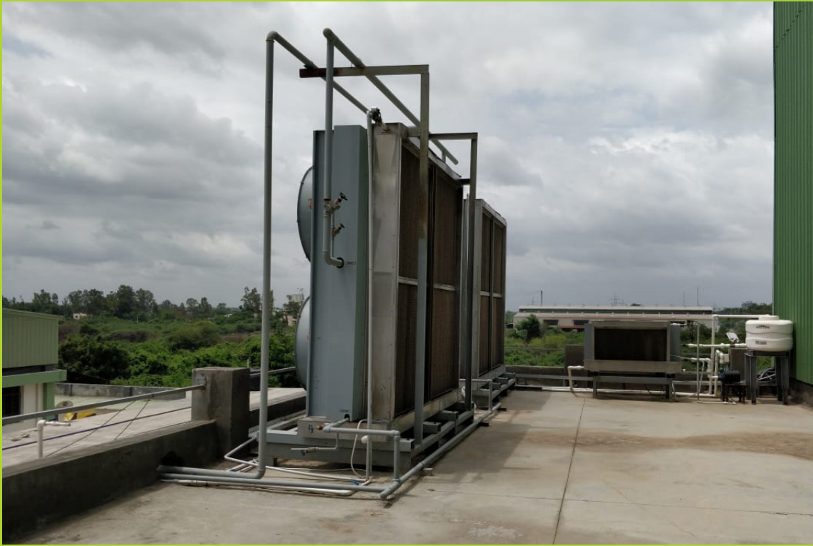
Air-Cooled Condenser with Adiabatic Precooling Pads (Left) and Dry-Cooled with Adiabatic Cooling Pads (Right)
