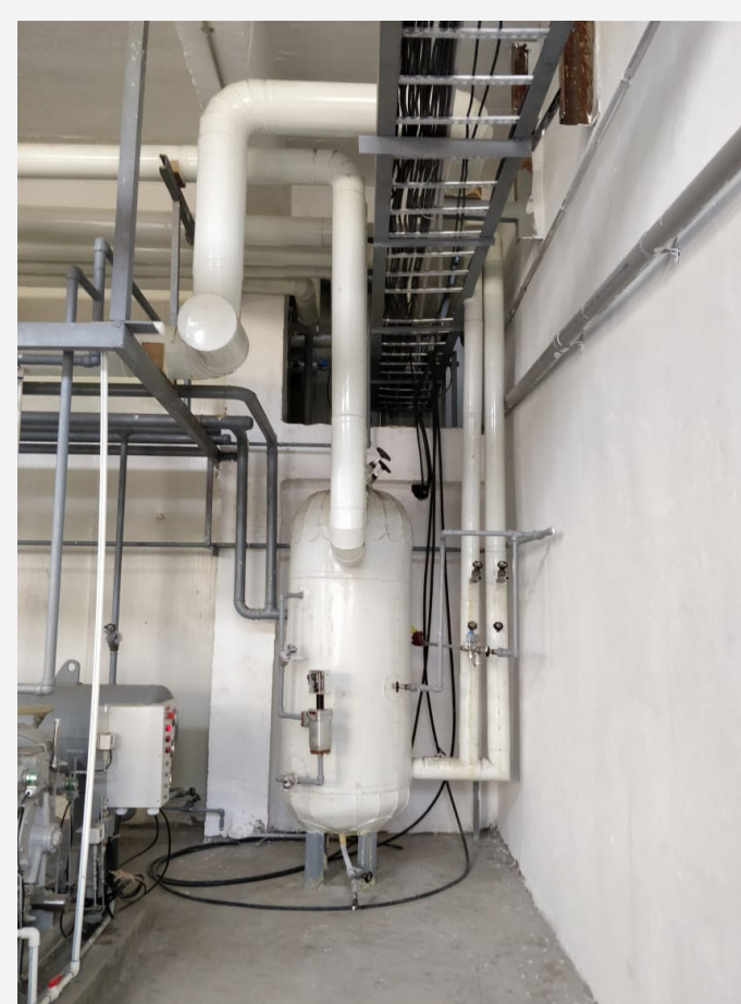
Intercooler in Machine Room
