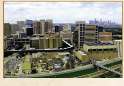
PHOTO 9 Thermal Energy Corporation (TECO), District Energy System, Houston, using stratified CHW TES. (courtesy TECO)
