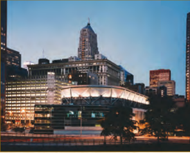
PHOTO 6 Northwind Ice Storage Plant, Chicago. (courtesy Enwave Chicago)
