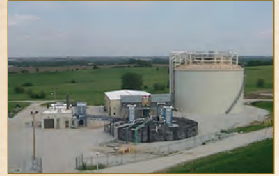
PHOTO 10 LES Peaking Plant with Ice TES for Inlet Air Pre-Cooling. (courtesy LES)
