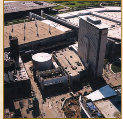
PHOTO 8 Trigen-Peoples McCormick Place Stratified Low Temp Fluid (LTF) TES, Chicago. (courtesy Chicago Bridge & Iron Co.)
