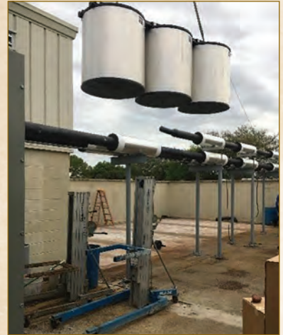
PHOTO 5 Ice Tank Installation at Brevard Schools, 2019. (courtesy Brevard Schools)
