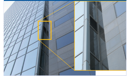
FIGURE 3 A building façade with features that camouflage additional OA louvers.
