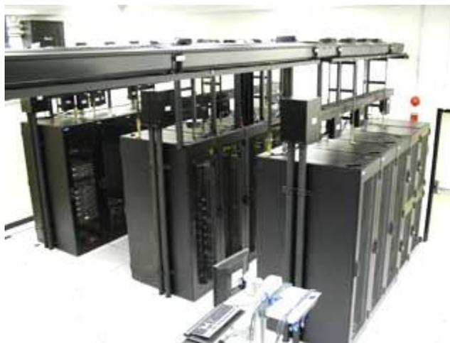
**Figure 23** Example of a modular busway system.
