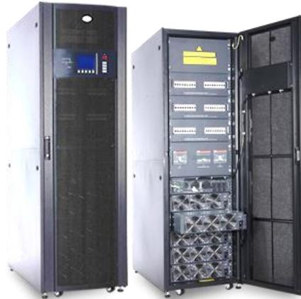
**Figure 13** Examples of smaller rack-based UPS units.
