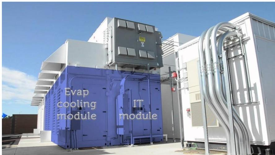
**Figure 5** Air-side economized modular data center with evaporative cooling module.
