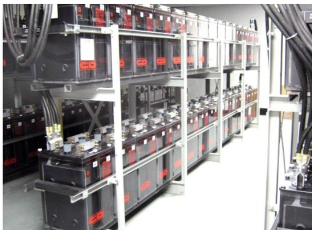
**Figure 15** Data center UPS battery room with flooded cell type batteries.
