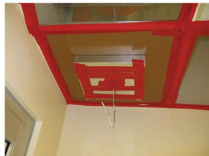
Test 1 Condition: Pressure Stabilizer (12"x12") is activated in operation. It is mounted on room ceiling which exposes to hallway. Door below also exposes to hallway when it opens.
