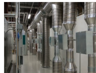
ABOVE Laboratory exhaust air valve arrangement emphasizes accessibility.
