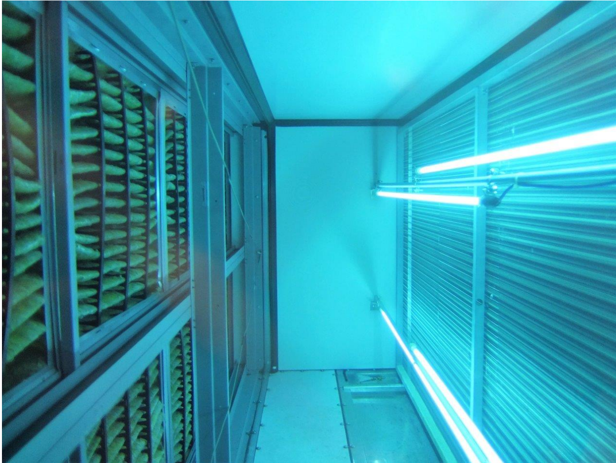
Downstream coil surface/air installation
