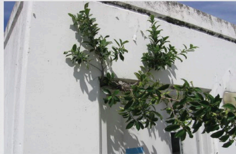
Figure 2.6-A Tree Sapling Growing from Upper Portion of Window Photograph courtesy of Phil Morey.
