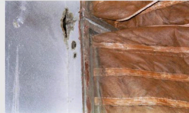
Figure 7.5-J Corrosion Penetration within an Air Handler
