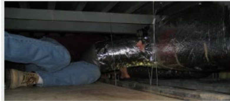
Figure 4.3-C System Location Limits Access
