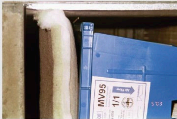
Figure 7.5-H Fallen Filter with Substantial Visible Gap
