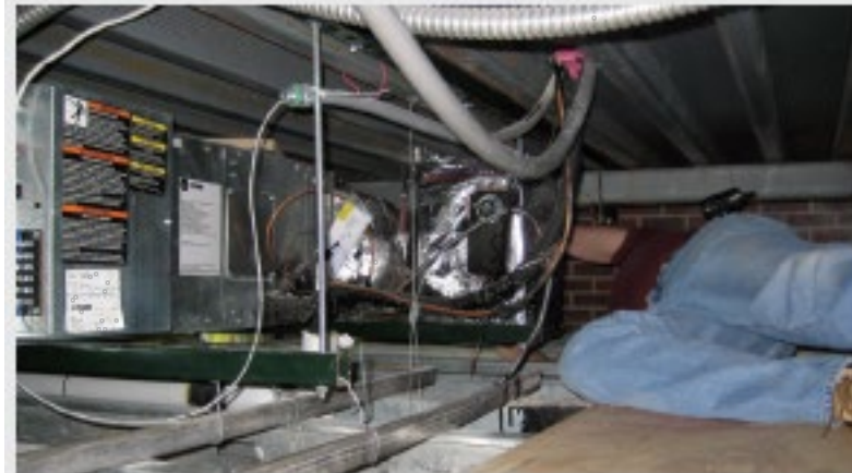
Figure 4.3-D All System Components not Readily Accessible
