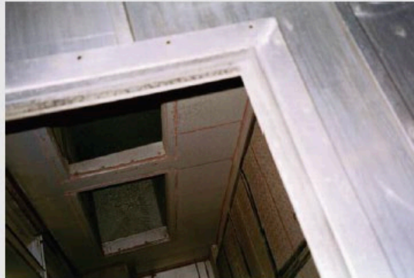
Figure 7.5-I Eroded Gasketing on Filter Access Door
