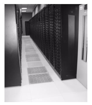
*Figure 2.70 Rack layout showing the cold supply-air row.*
